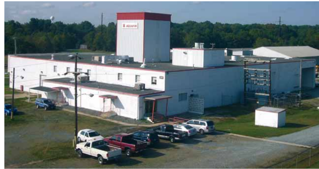
AQUAFIN Inc. plant in Elkton, MD, USA
