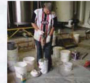
Mixing VAPORTIGHT COAT®-SG in supplied container.
