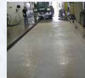
Finished surface, ready to receive top-coating.
