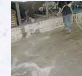
Cleaning/rinsing surface from debris.
