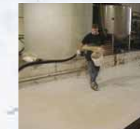
VAPORTIGHT COAT®-SG2 only: Application step 4, sanding of surface for bonding of subsequent epoxy top-coating.
