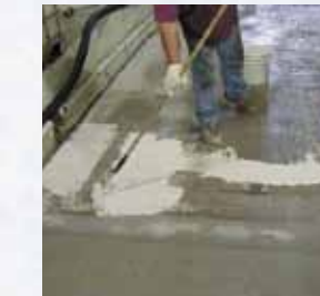
SG2 & SG3: Application step 1, spreading material evenly over surface with squeegee or roller.
