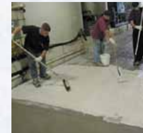
SG2 & SG3: Application step 2, scrubbing material into the substrate pores with a brush. Application step 3, back-roll with a shortnap, non-shed roller to achieve a uniform finish.
