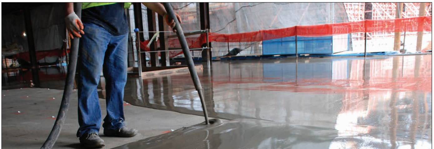
AQUAFIN LEVEL-Ultra is moisture tolerant, allowing for applications before buildings are enclosed.
