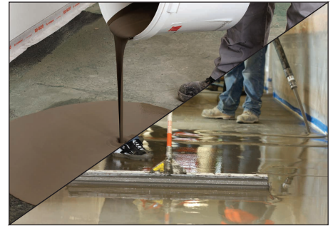
AQUAFIN LEVEL-Ultra has great healing and flow characteristics and can be barrel mixed or pumped.
