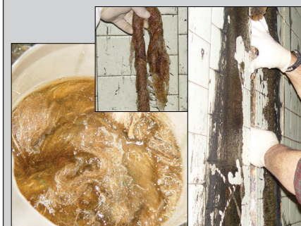
Typical application of Oakum in a leaking joint.
