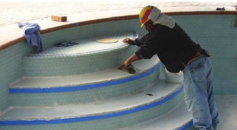
Since tiles and pool plaster are not waterproof, a waterproofing membrane should be used beneath them to extend the service life of the pool.
