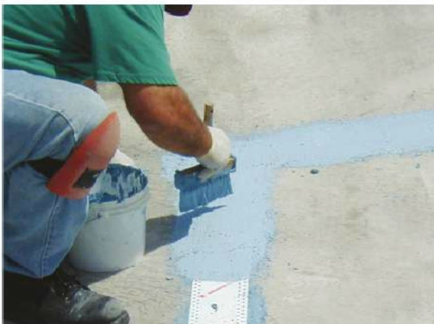
Joint tape is used to reinforce wall/floor joints (top) and to repair cracks prior to applying the waterproof coating.
