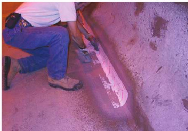
Since tiles and pool plaster are not waterproof, a waterproofing membrane should be used beneath them to extend the service life of the pool.
