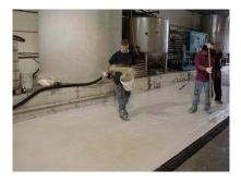
10. Immediately broadcast sand to rejection (full broadcast) on top of fresh SG2.
