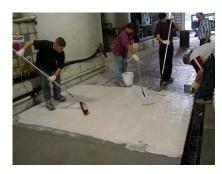
8. Carefully scrub SG2 into the pores with a long handled broom or scrub brush.
