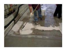
7. Pour appropriate amount of material onto slab and spread evenly with a roller or squeegee.
